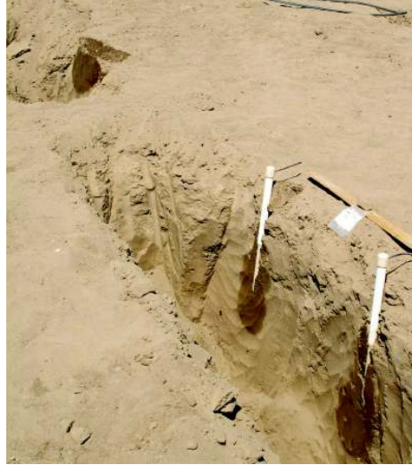
Figure 12. View of surface drip (left) and Deep Drip™ (right) wetting patterns along Drip Line 2 (west locations)
