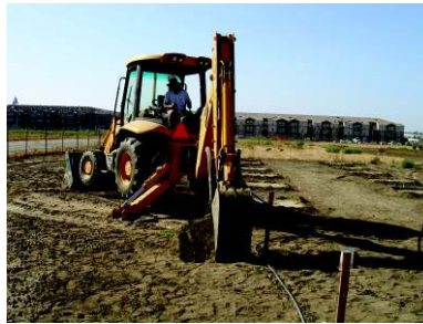
Figure 7. Backhoe used to dig trench at each testing location
